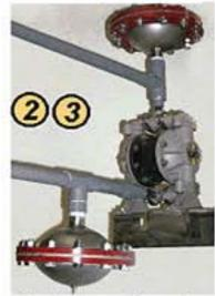
Single connection pulse dampers are also available , but flow-thru is standard single connection is more costly. You can always take a 2 connection and use one. & the other for system drain
